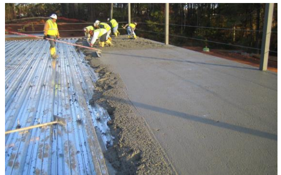
Composite Steel Deck
